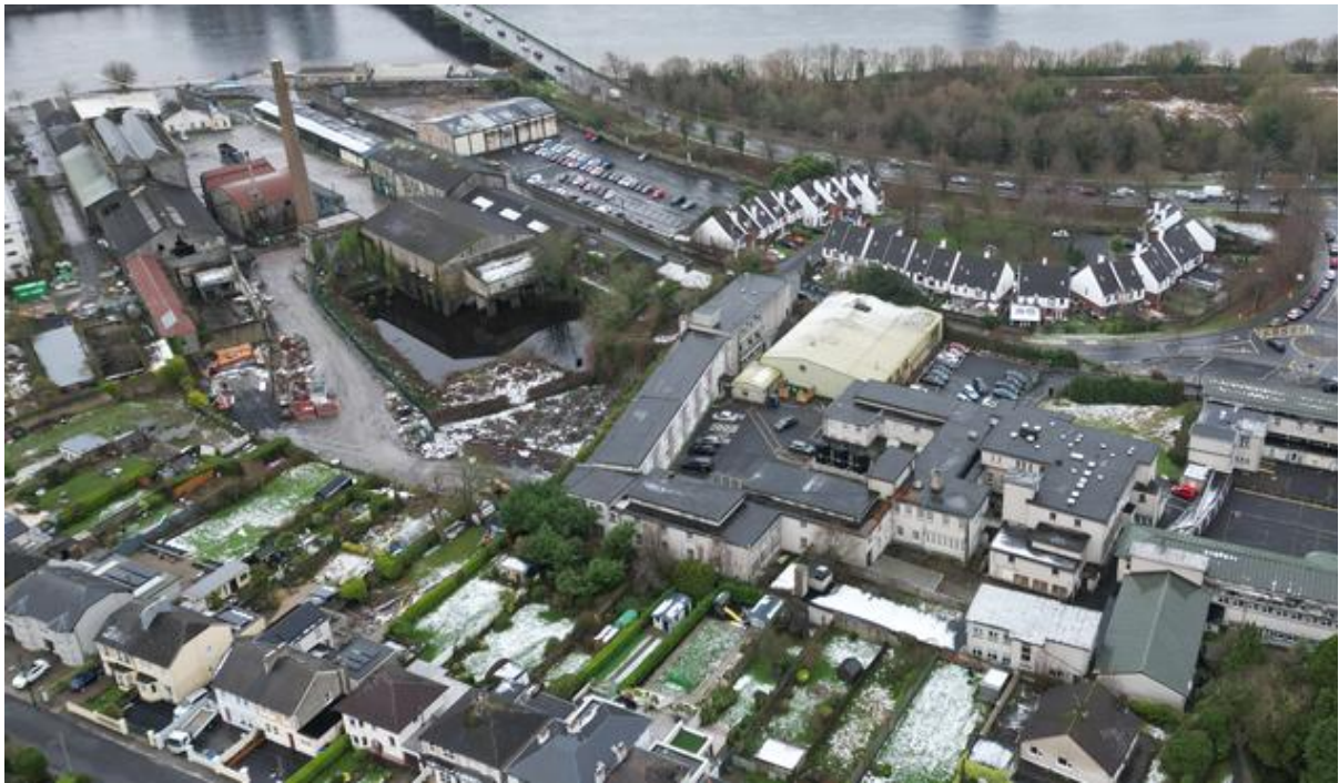
Plate 8.4: Drone view of site 10/1/25 (from NE)
