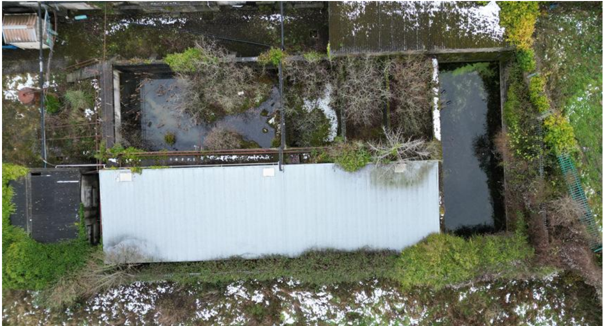
Plate 8.31: Vertical drone view of Upper Reservoir (W to top)
