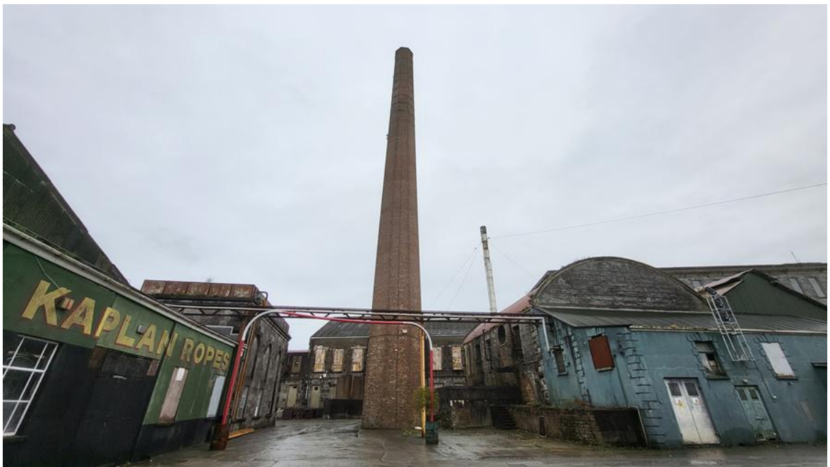
Plate 8.12: Chimney Stack (from W)
