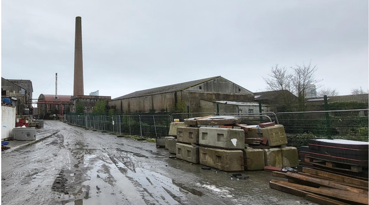
Plate 8.19: Engine House (from NE)
