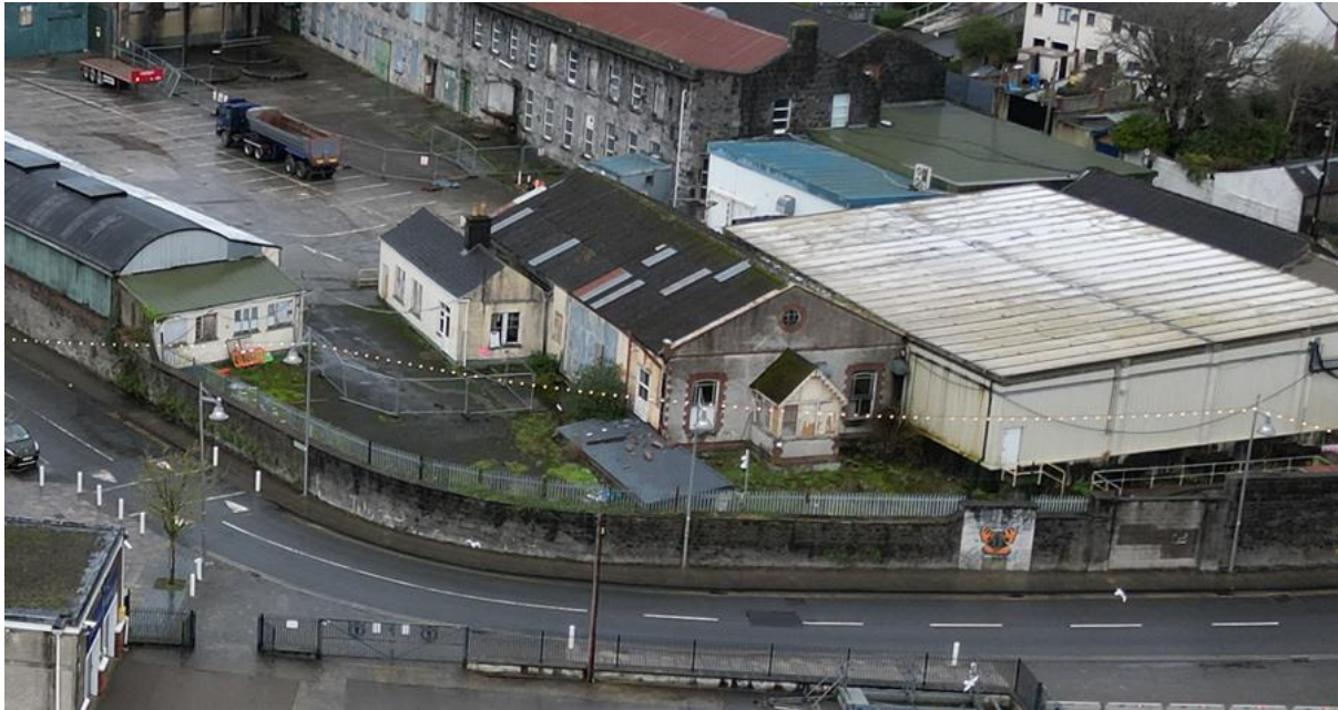
Plate 8.27: Drone view of Offices and Warehouses (from SSW)
