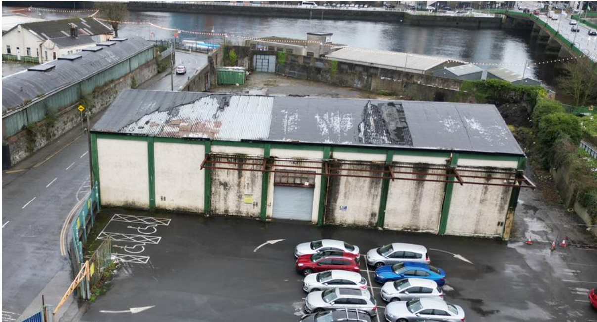
Plate 8.33: Drone view of South Warehouse (from NNW)
