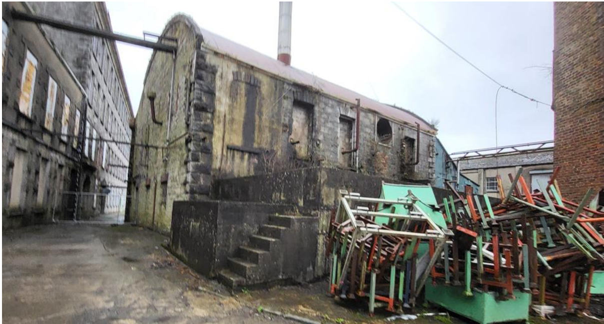
Plate 8.15: Engine House (from NNE)
