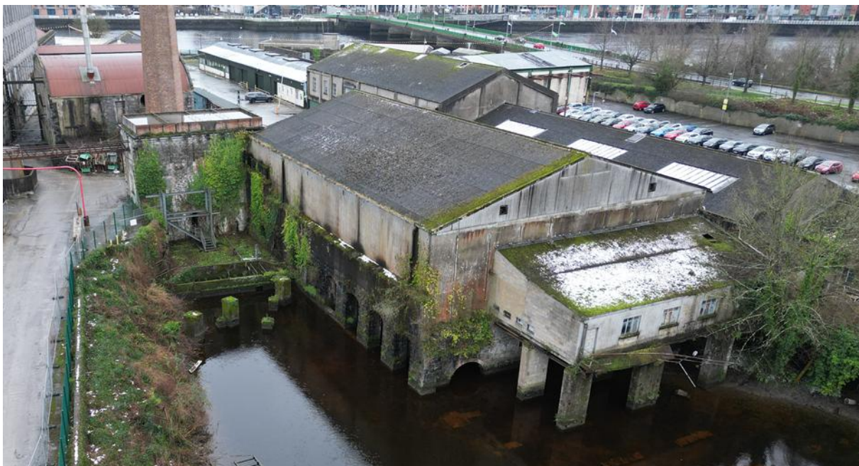
Plate 8.18: Drone view of Engine House (from NE)
