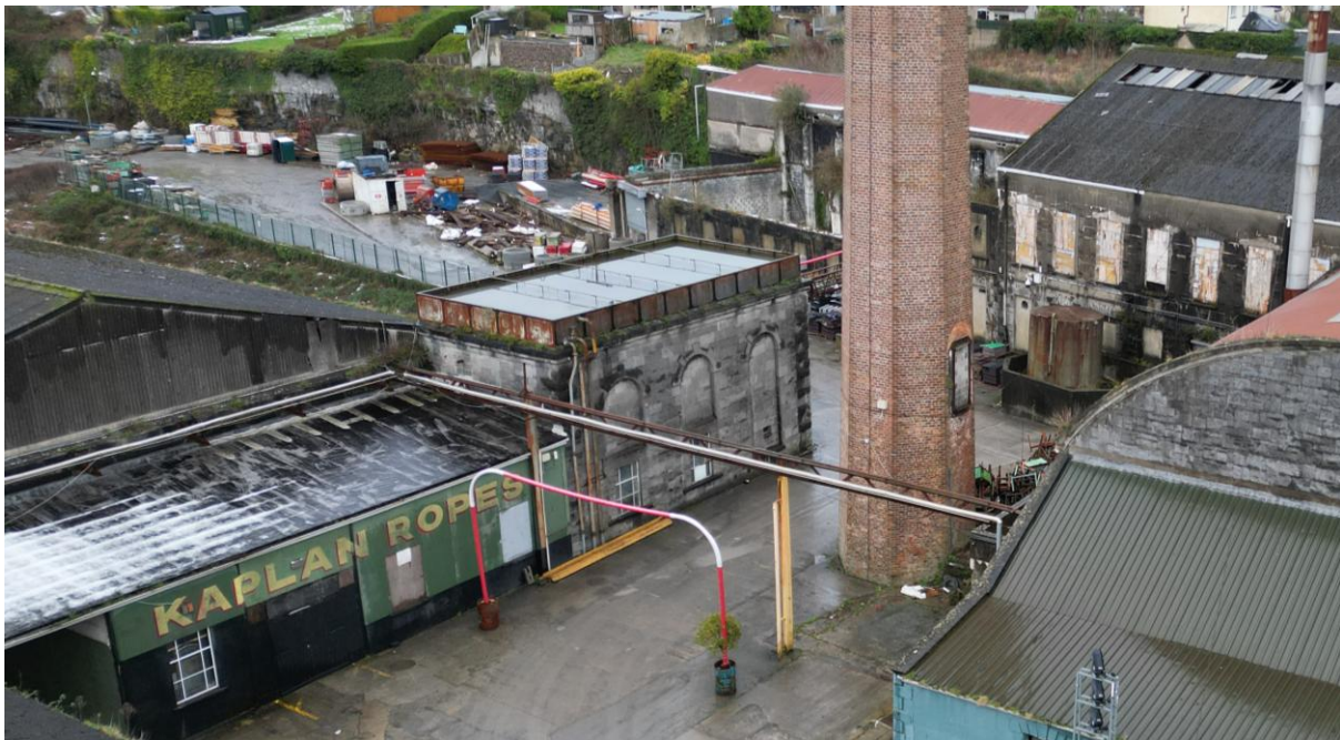
Plate 8.16: Drone view of Water Tank Building (from SW)
