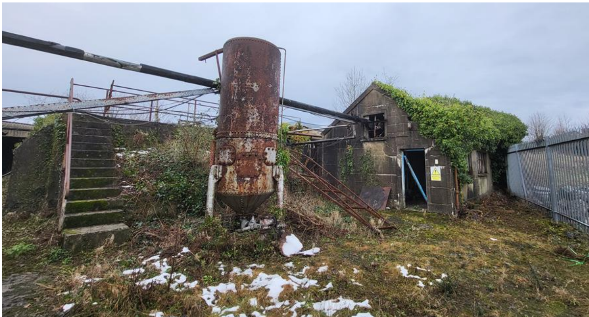
Plate 8.32: Upper Reservoir (from SW)
