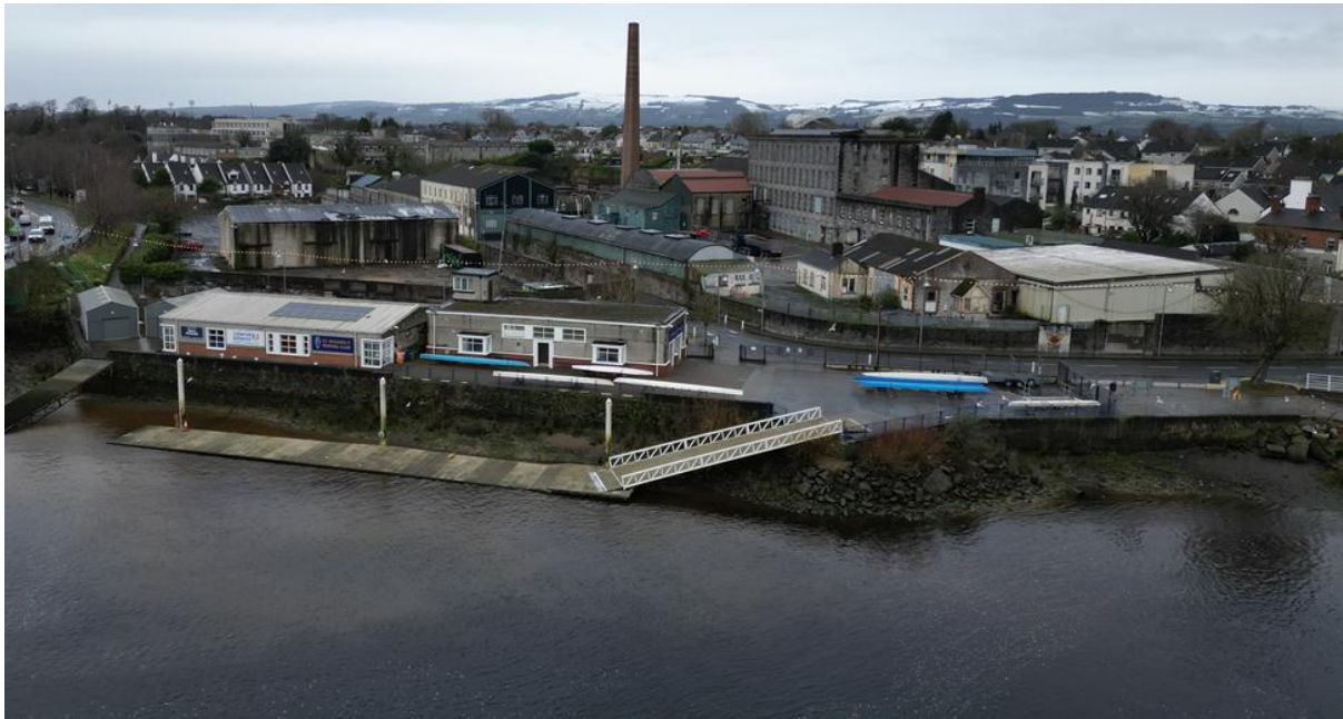
Plate 8.41: Drone view of Rowing Club (from SSW)
