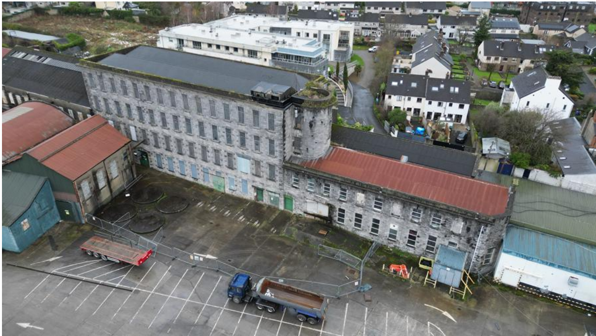
Plate 8.8: Drone view of Flax Mill (from WSW)
