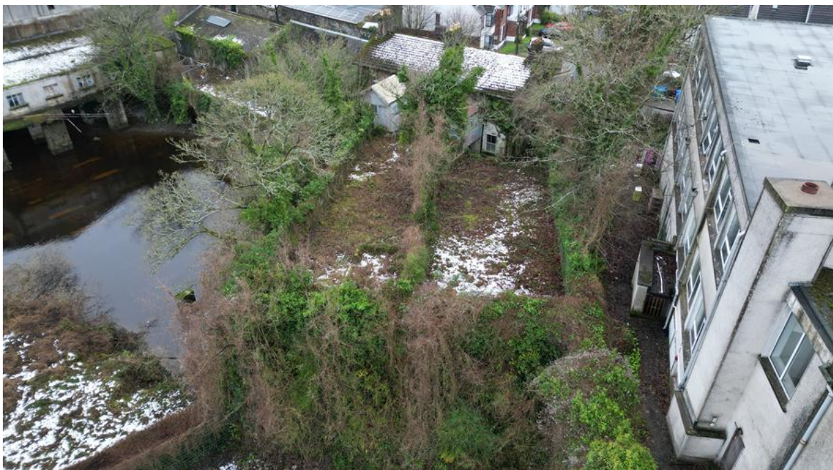
Plate 8.36: Drone view of Victorian Terrace (from ENE)
