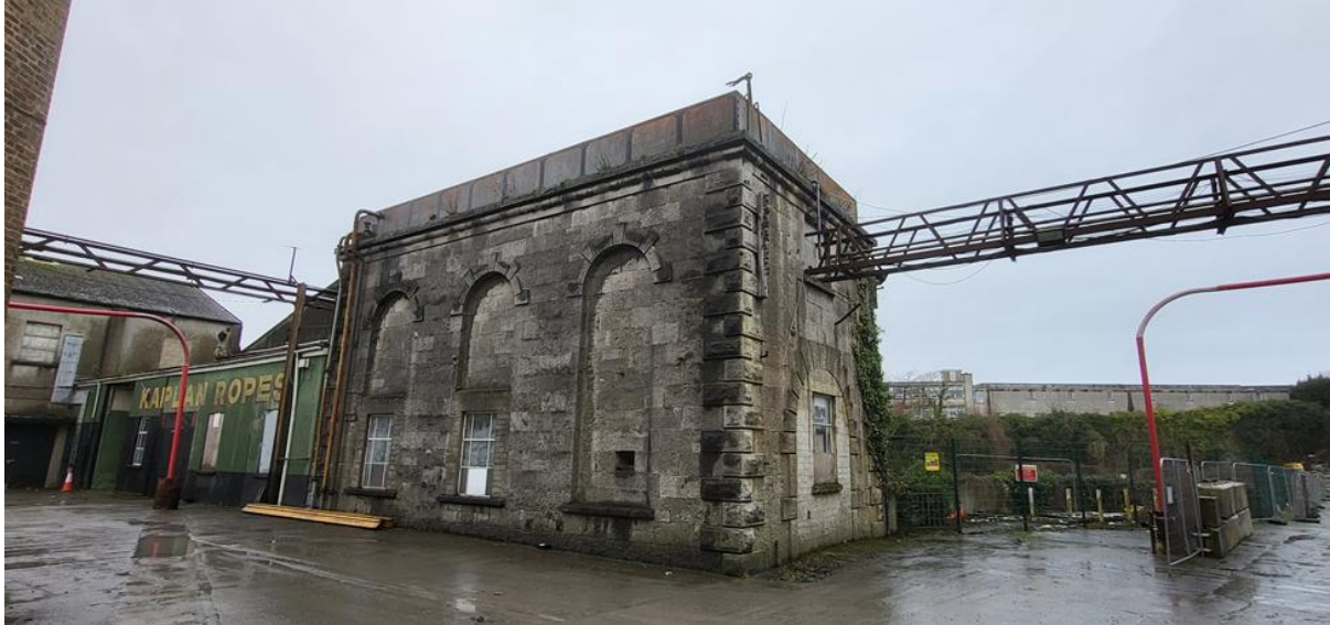
Plate 8.17: Water Tank Building (from SE)
