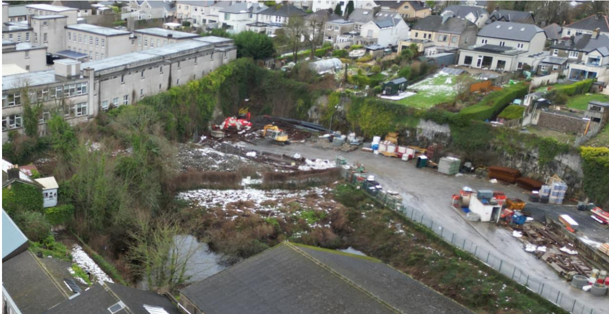
Plate 8.37: Drone view of Quarry Face (from SW)
